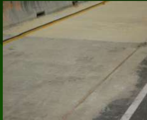
•Replacement HOV lane at I-10, Los Angeles, CA, 2009 (12-hrs RSC)
