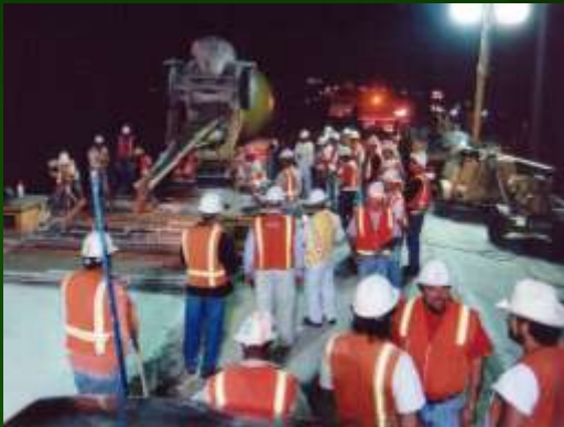
•Pavement replacement at I-10, Pomona, CA, 2009 (4-hrs RSC)
